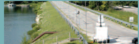
California has hundreds of state-regulated High-Hazard Potential dams that need EAPs. Many are in suburban areas.
