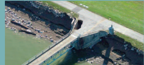
Lake Livingston's EAP was triggered when Hurricane Rita tore away rip-rap and caused extensive damage.
